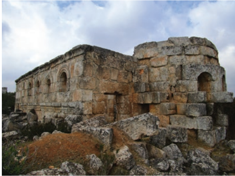
General view from the southeast showing the apse and the southern facade
