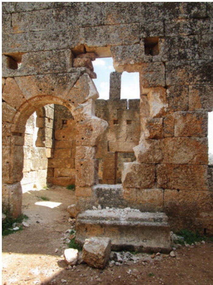
Figure 5. Deir Sobat, collapsed part of interior wall
