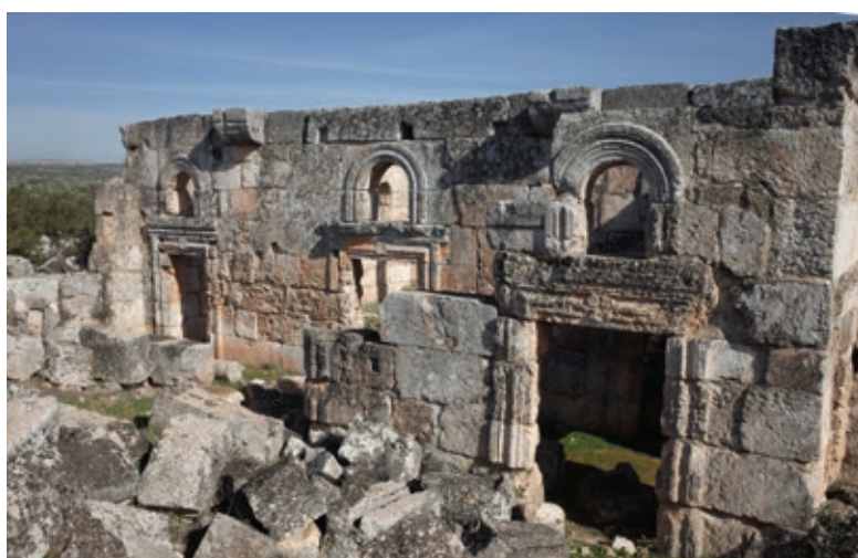
General view from the west
