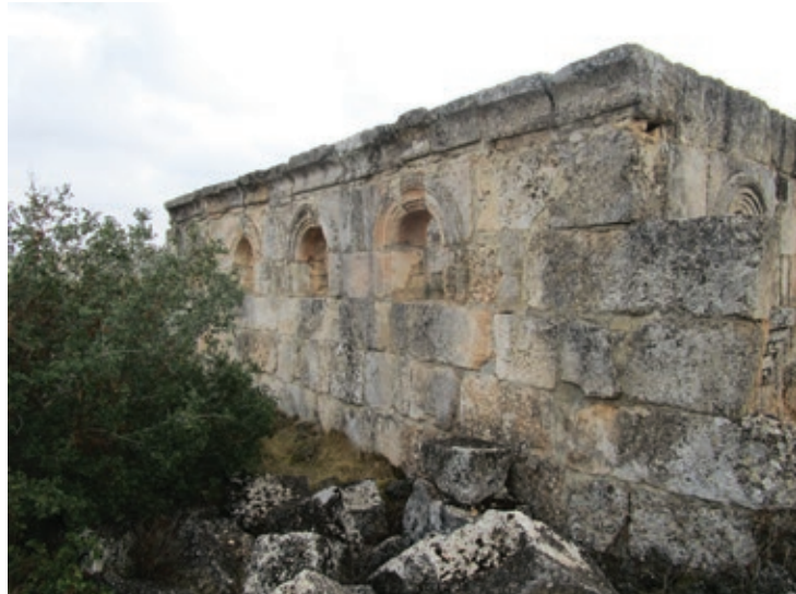
General view from the northwest showing northern facade
