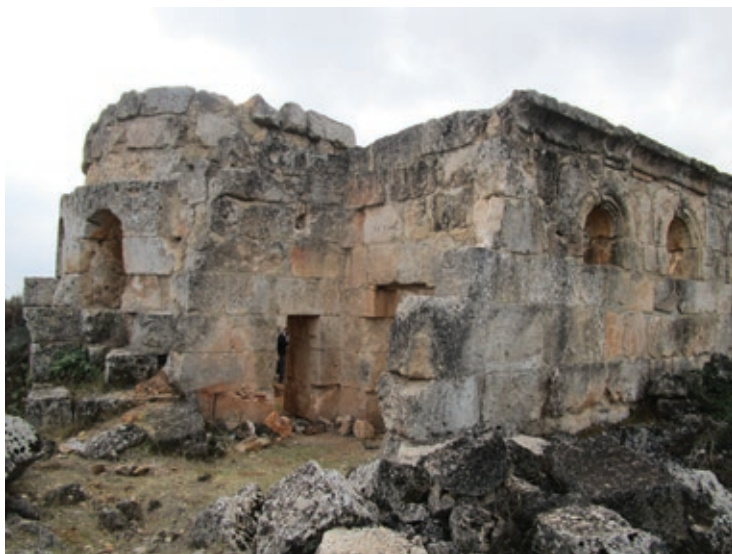
General view from the northeast
