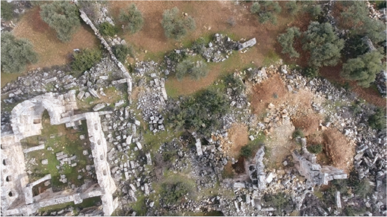
Figure 11. Church 4, illegal excavations and destruction near by
