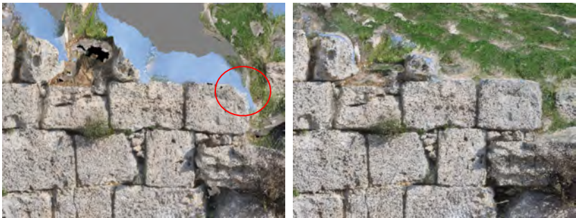
Figure 13. The image on the left is corrupted due to lack of photography from above. The image with additional photograph from above gives a better model.
