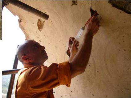
A soft grouting mortar was injected between the rock support and the earthen rendering.
