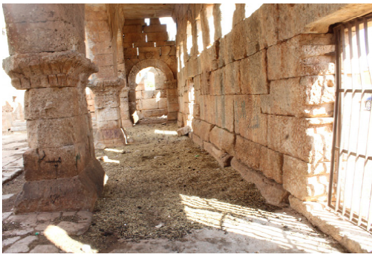
South side aisle
