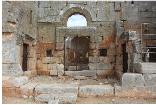
Main western entrance
