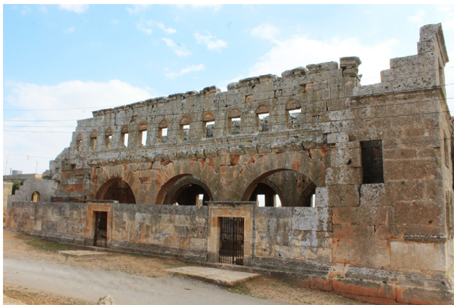
Northern side facade showing two doors and northern wall arches
