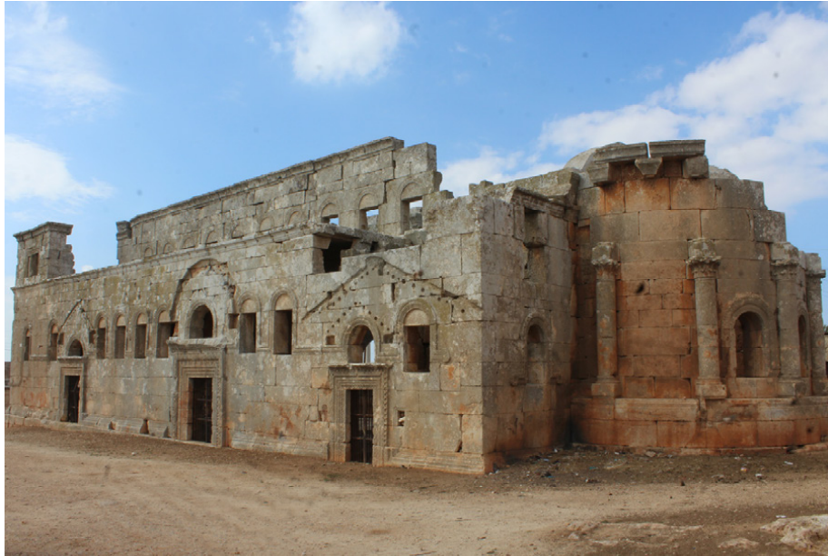
Southern side facade showing three decorative doors
