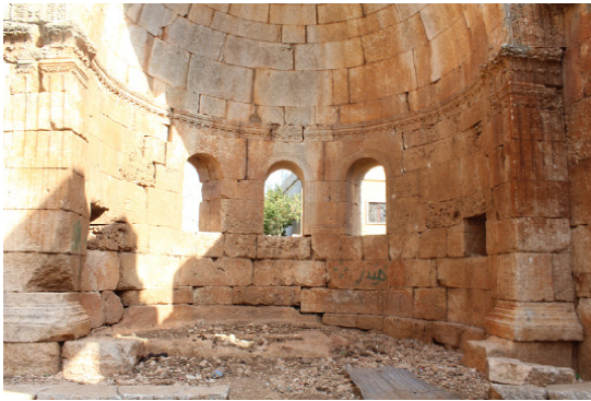
Apse (interior part)
