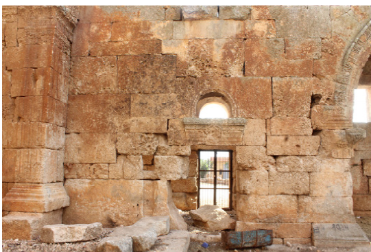
Southeast side room entrance
