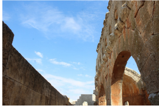
North side wall
