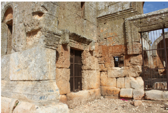
Left side square tower (down)
