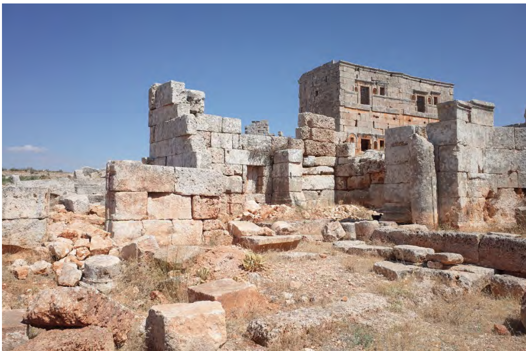
Interior north eastern facade
