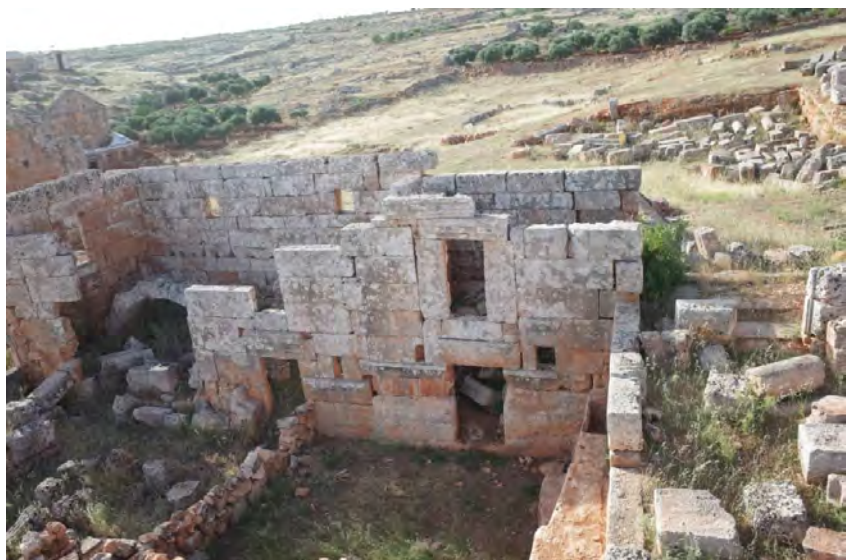
Figure 2 The current condition of Serjilla's buildings
