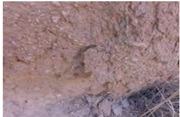
Figure. 1.4 Condition of area treated with Permeate HS-360. The lower portion showed weathering under the consolidated layer (Sep 2016)
