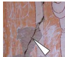
c. Structural cracking
