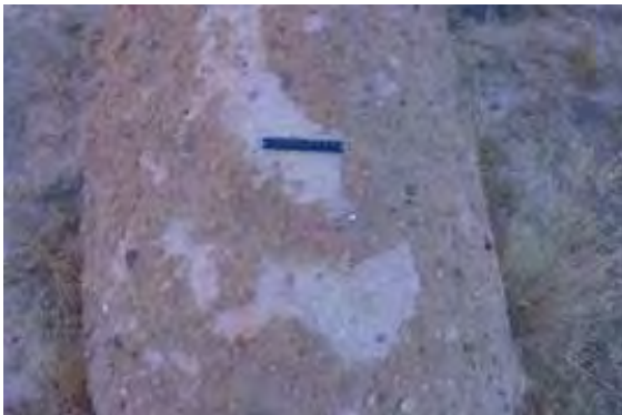
Figure. 1.3 Condition of area treated with Permeate HS-360. Some areas of the consolidated surface were detached (Sep 2016)
